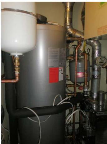
Vitocell-B CVB Dual Coil Storage Tank(80gal)
