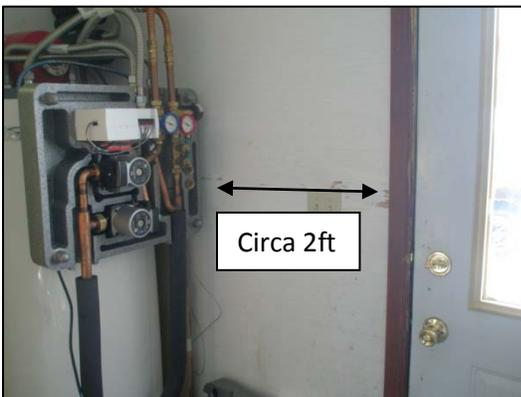
Pro-lite controller and Hilio-pack pro heat exchanger with Wi-Fi and data logging. (uncovered)
