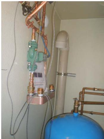
Auxiliary pump and flat plate heat exchanger for hydronic base board heating loop.
