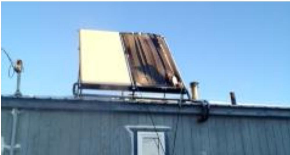
Picture 2: Wind damaged Heliodyne flat plate collector
