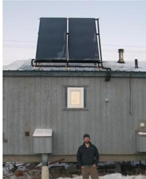
Heliodyne Flat Plate Solar Collector.
