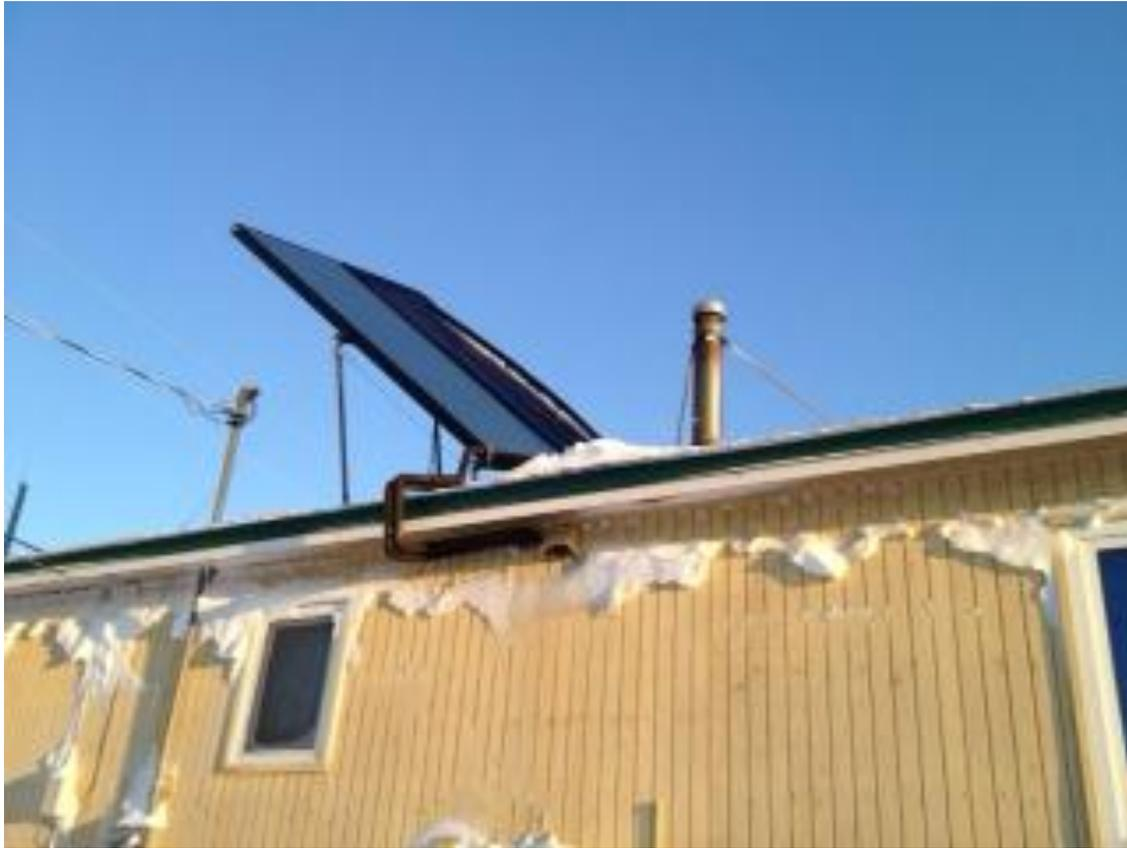
Picture 1: Wind damaged Heliodyne flat plate collector
