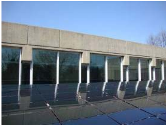
Princeton University E-Quad Solar Array Installation
