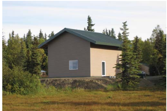
Figure 1. A view of the house from north west. Yes, it does have a window on the north side — not a good idea for passive solar design, but we couldn't resist putting one there because of the beautiful mountain view towards the north. The majority of our window area is in the south wall. The house has outside dimensions of 24' x 24', 1½ stories (main floor plus a loft), two bedrooms, one bathroom, and is located in Dillingham (about 11,000 heating-degree-day climate).
