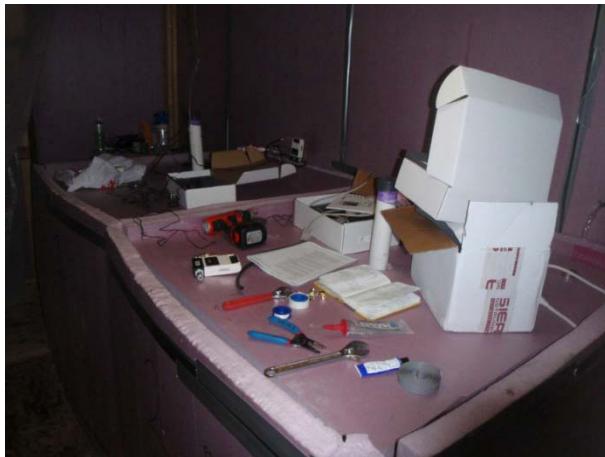
Materials for installing flow meters.
