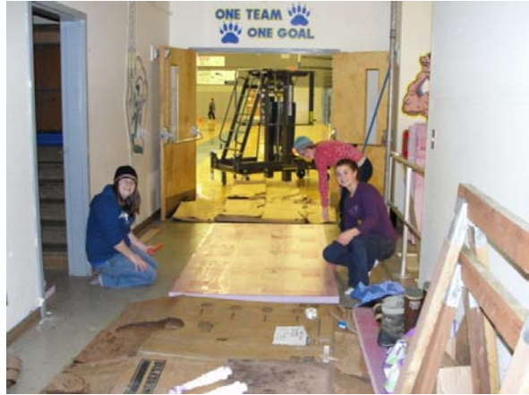
Students prepare insulation panels to fit around primary slurry tanks.
