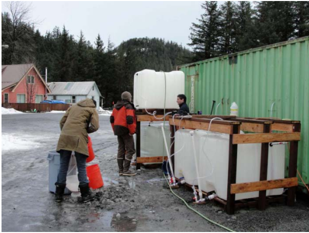
McFadden, Shaw, and Culhane place fittings on water pressure systems.
