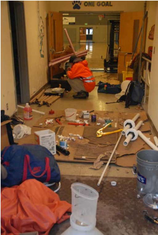
Peter Anthony prepares construction materials.
