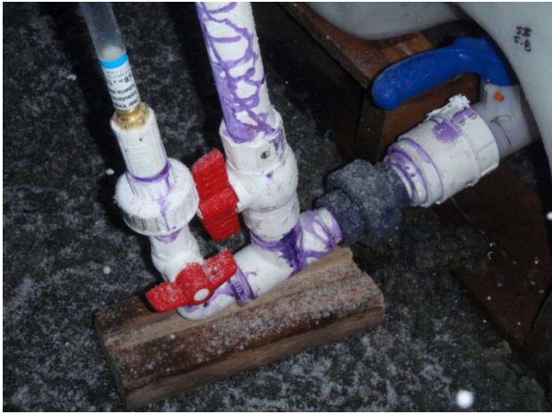
Working with water transport pipe fittings while snowing (Jan. 2010).
