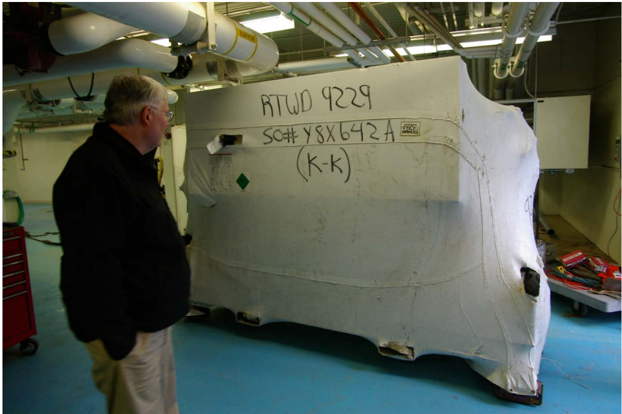
Figure 2 Installing first Trane heat pump in ASLC boiler room - March 17, 2011
