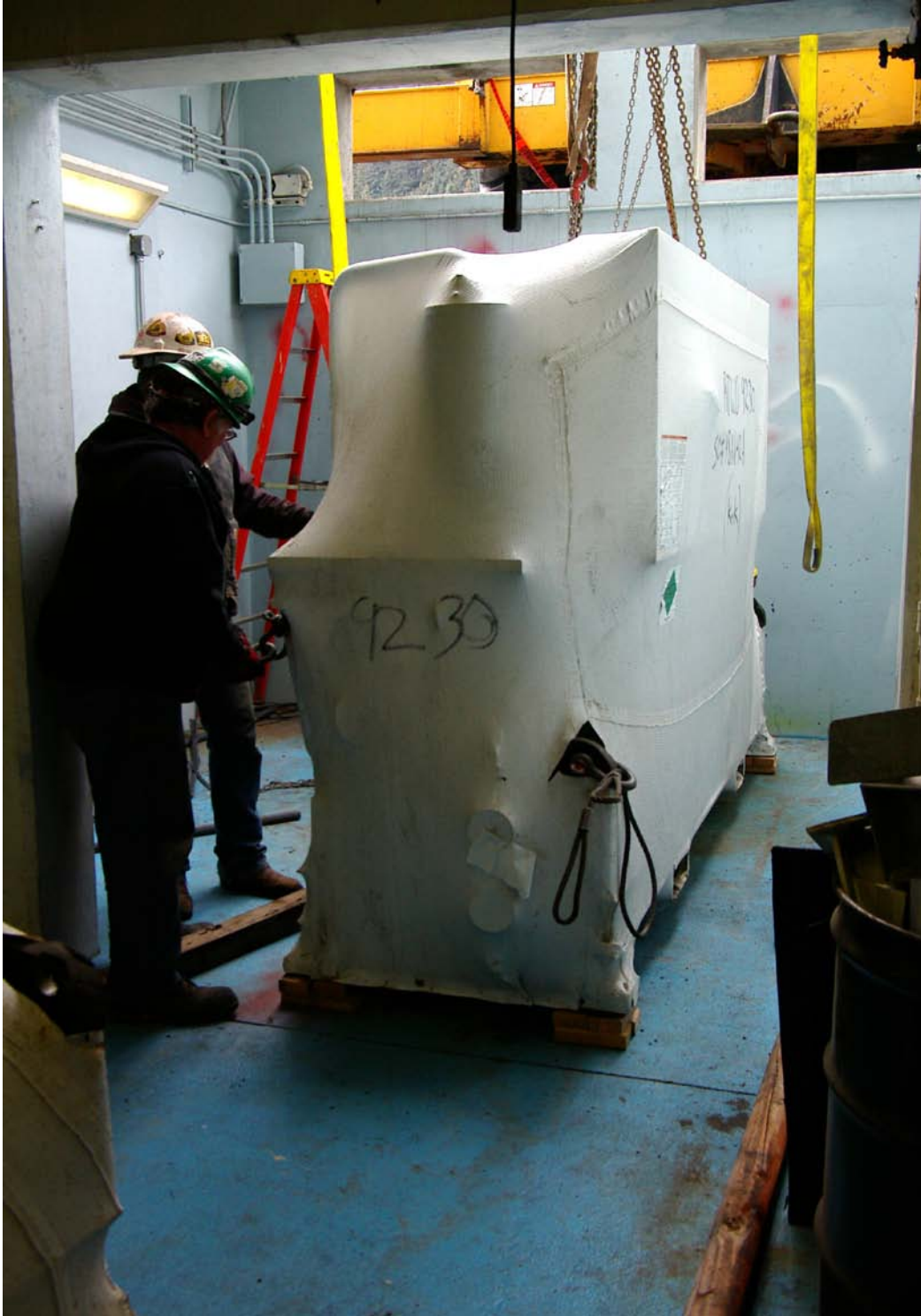
Figure 4 Installing second Trane heat pump in ASLC boiler room - March 17, 2011
