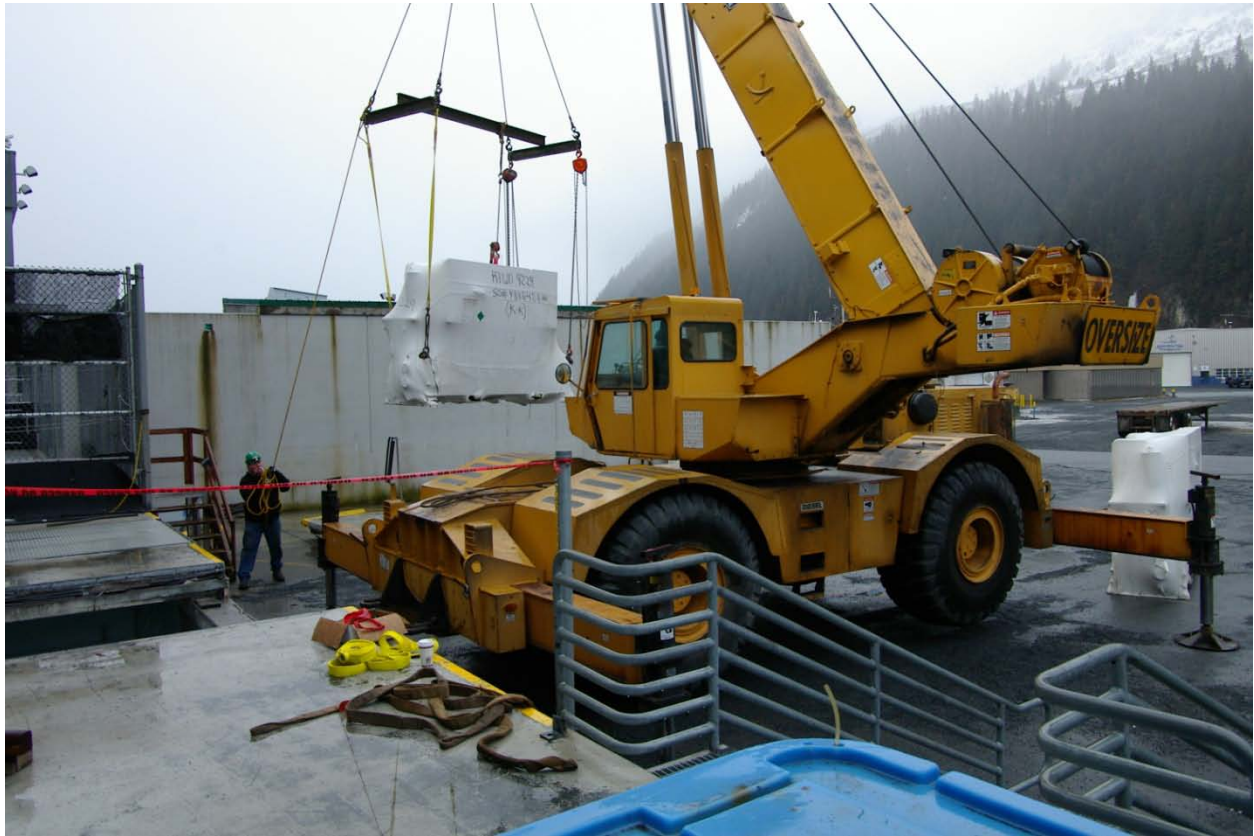
Figure 1 Installing first Trane heat pump into ASLC boiler room – March 17, 2011
