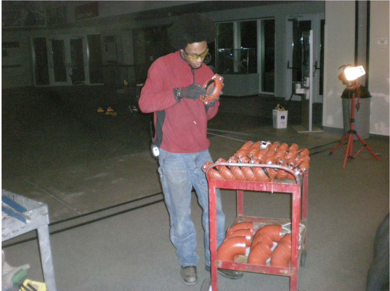
Figure 9 ASLC LSS Technician Isaac London preparing Victaulic couplers for installation - April 5, 2011
