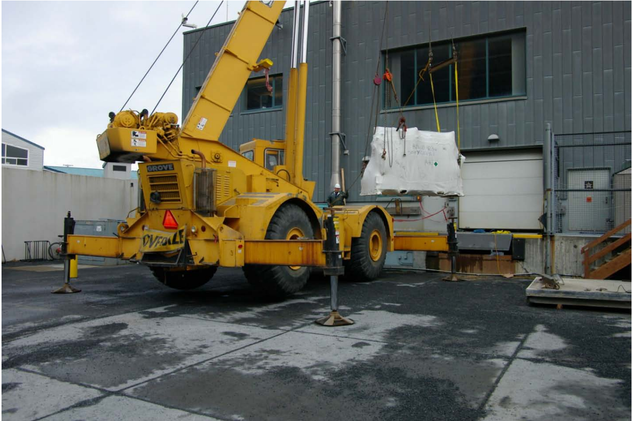
Figure 3 Installing second Trane heat pump in ASLC boiler room - March 17, 2011
