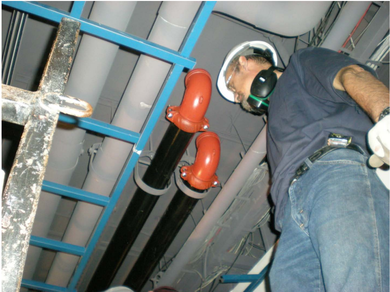
Figure 6 ASLC Facilities Technician Dan Rice installing Victaulic heating loop piping - April 4, 2011
