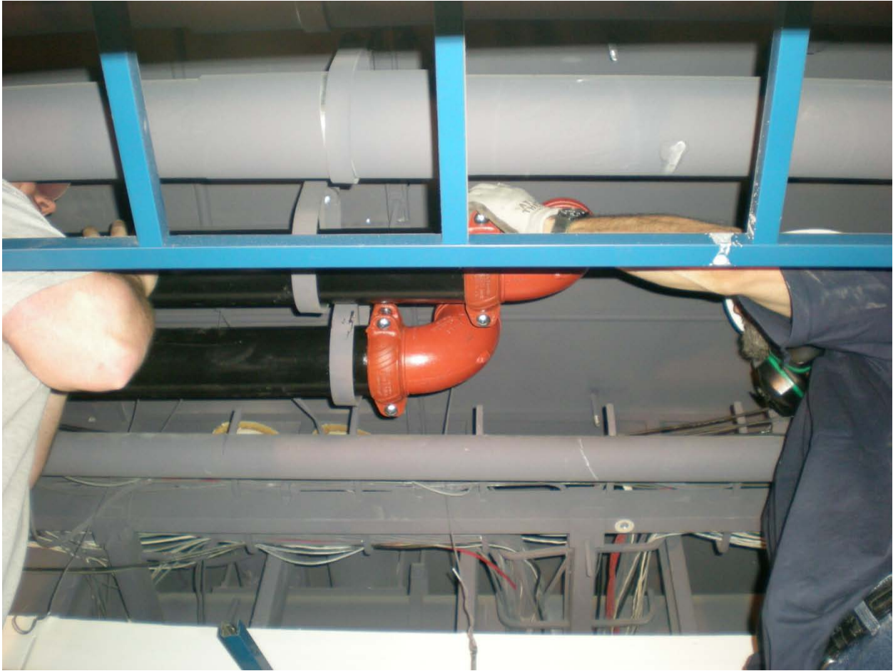
Figure 7 ASLC Building Maintenance staff installing Victaulic heat loop piping - April 4, 2011
