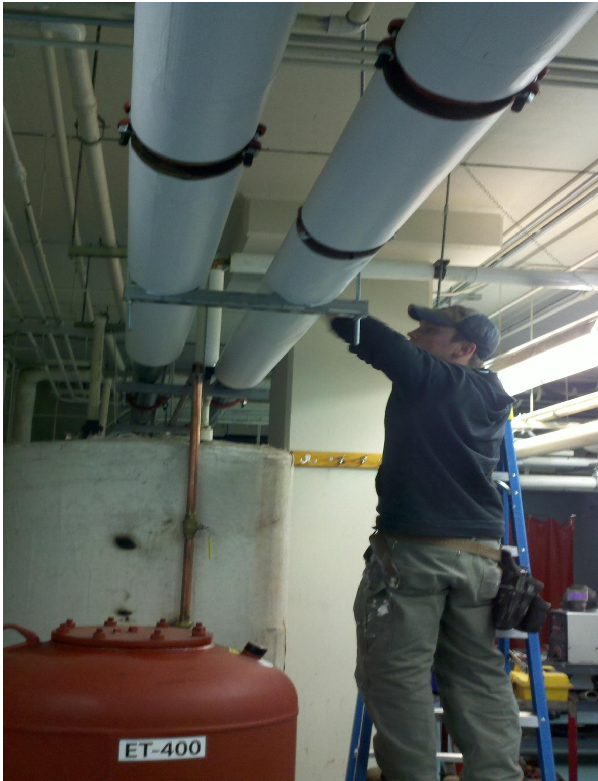
Figure 1 Installing pipe insulation
