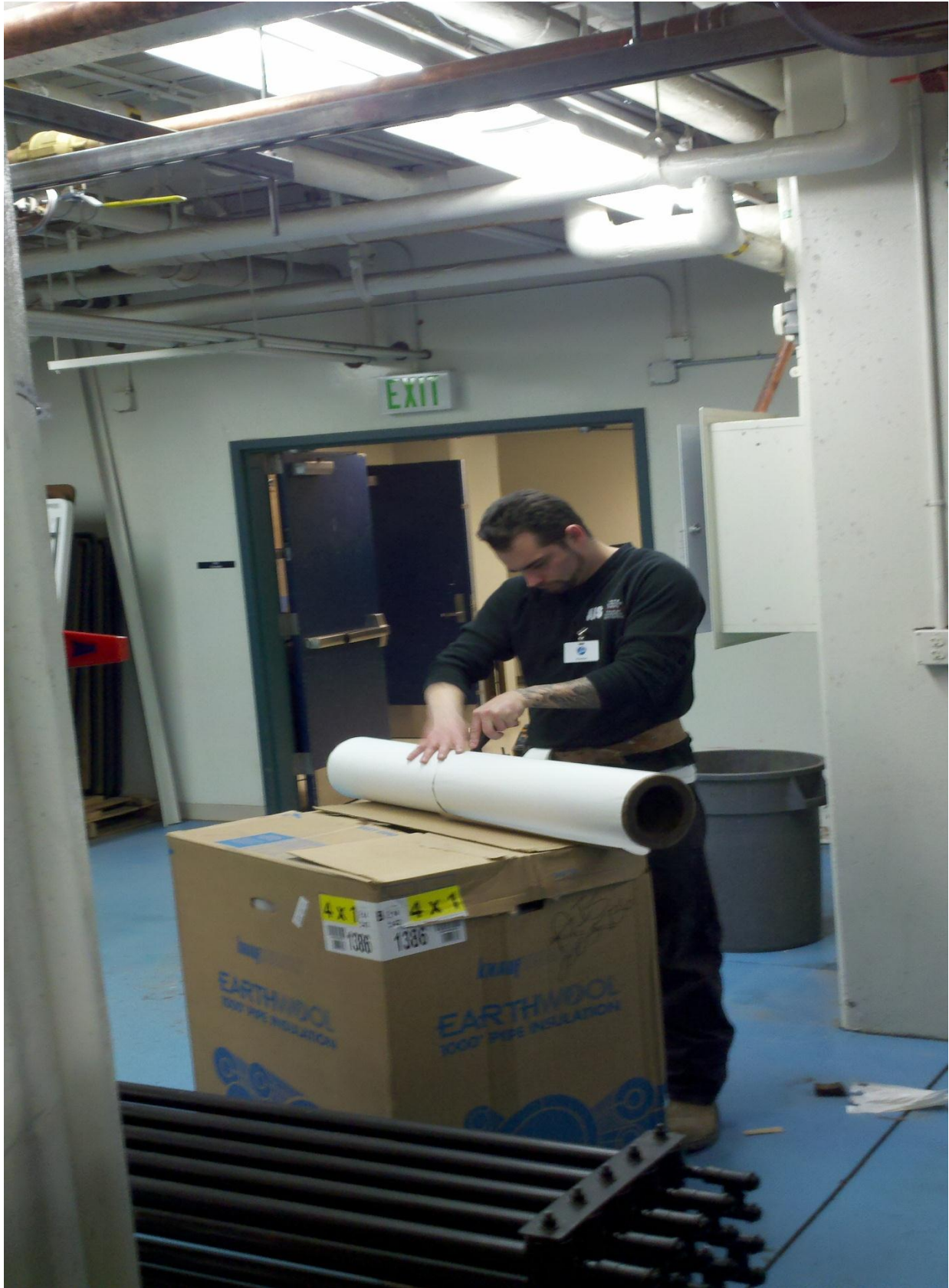
Figure 4 Installing pipe insulation
