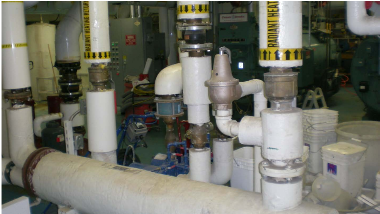
Figure 10 Pavement Heating Heat Exchanger
