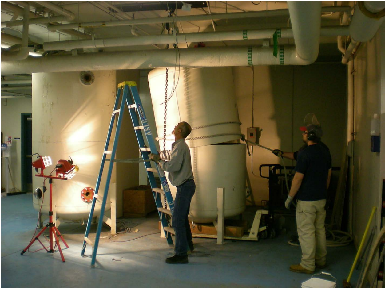
Figure 1 Removing Culligan System Tanks
