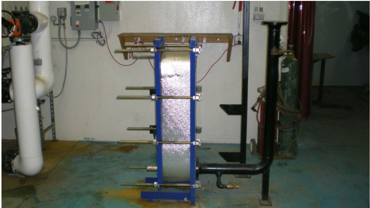
Figure 3 Removal of Salmon Project HX - Location of Seawater HP HX 6
